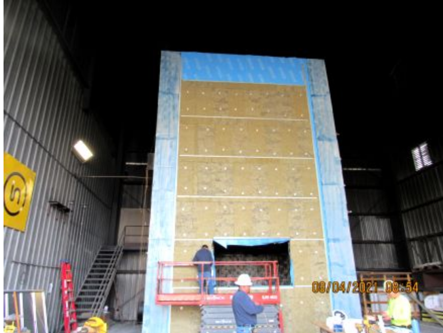
Photo No. 5 Insulation installed
