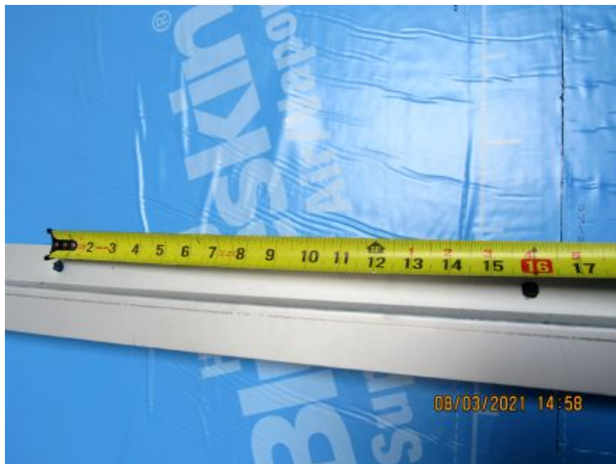
Photo No. 4 Z girt attachment spacing
