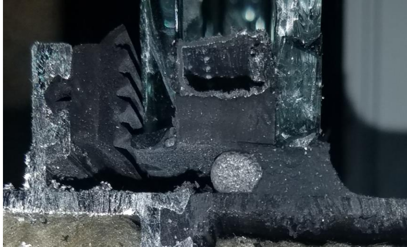
Glazing gasket and backer rod with silicone
