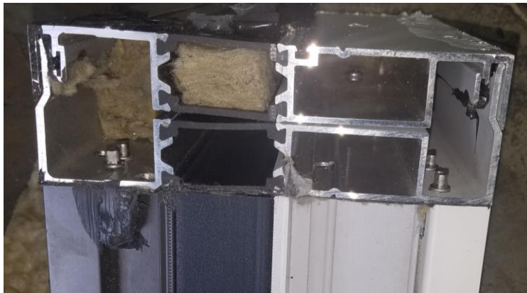
Frame corner joint
