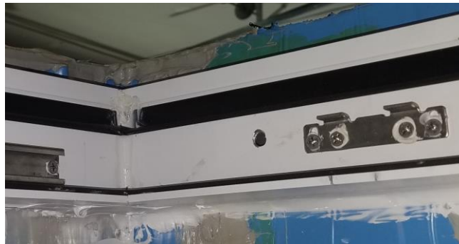
Top keeper and vent hole
