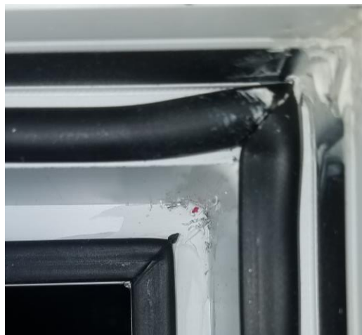
Frame weather-stripping corner
