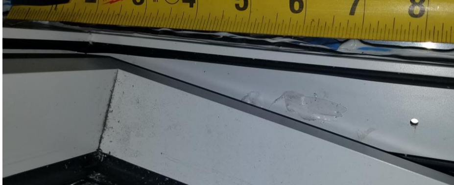
Venting hole in the sill
