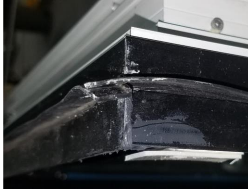
Sash corner weather-stripping corner
