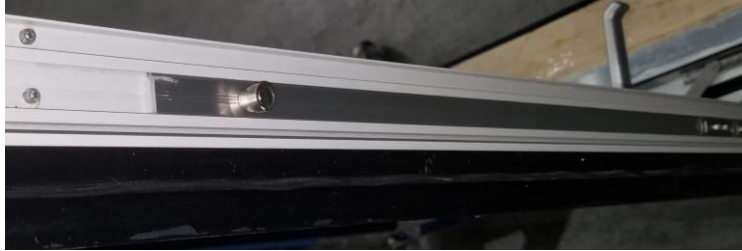
Multi-point locking bar
