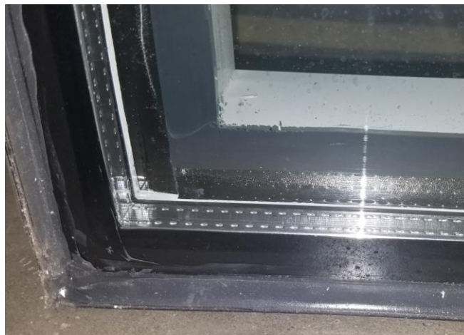
Exterior glazing silicone
