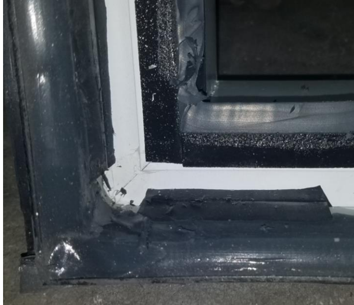
Exterior glazing silicone and interior glazing tape and silicone
