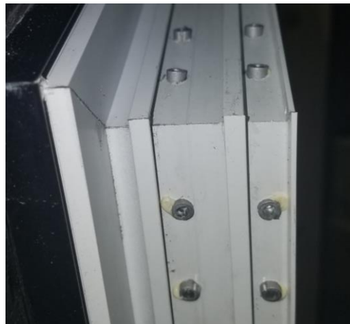
Sash corner joint rivets
