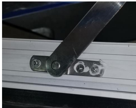
Sash limiter on the sash
