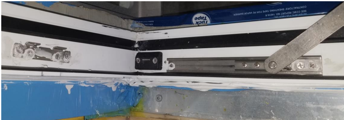
Sash limiter, riser block and bottom keeper
