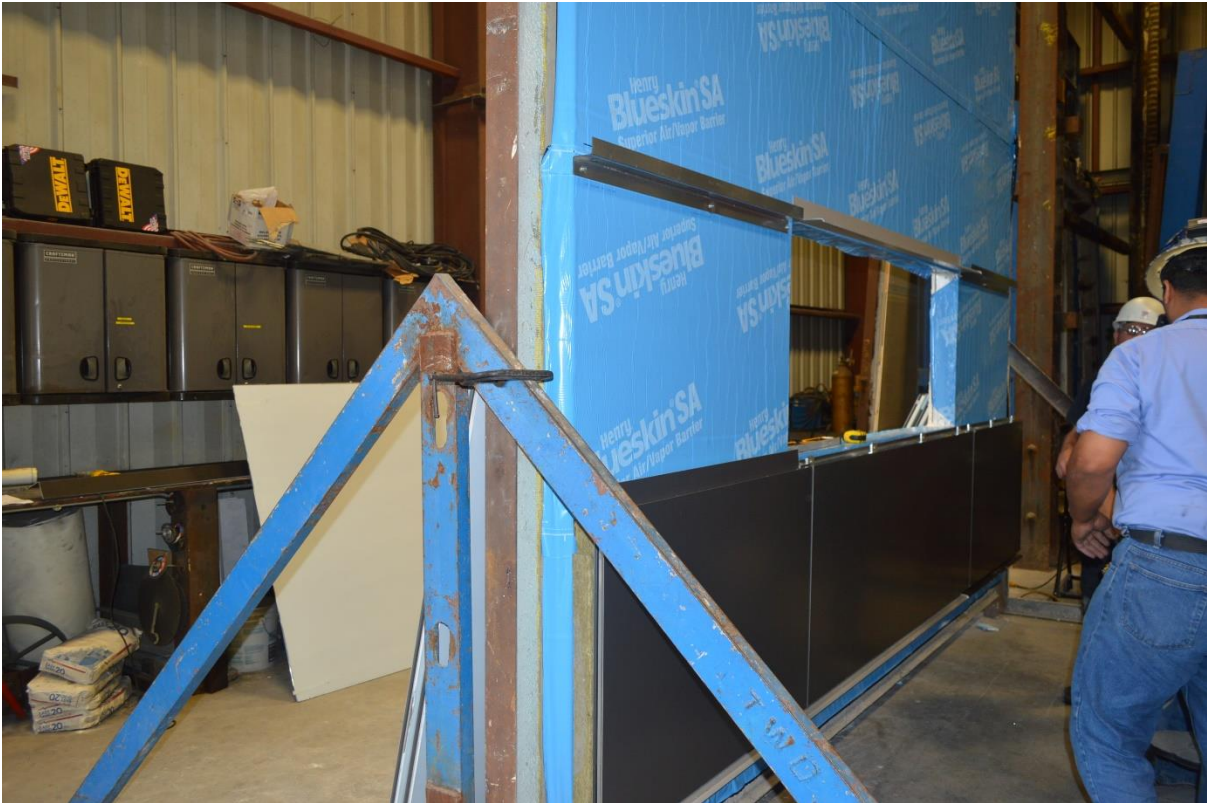
Figure B-3. Aluminum Composite Panel Installation.
