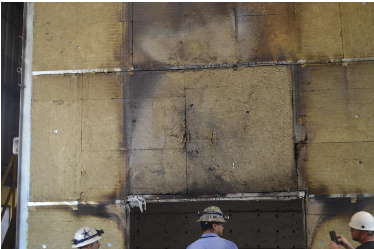
Figure B-18. Mineral Wool Insulation after Fire Exposure.
