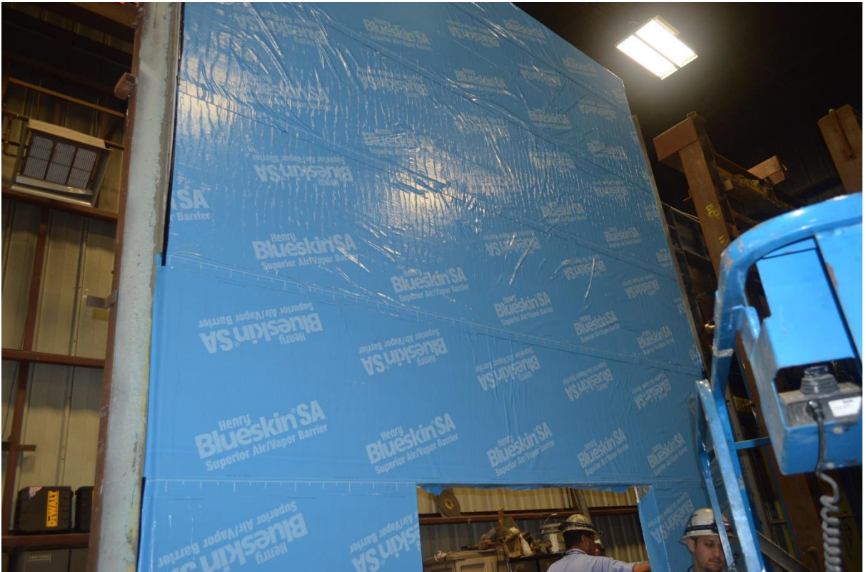
Figure B-2. Installation of Blueskin® SA Air and Vapor Barrier.
